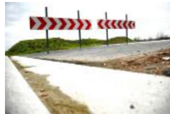
Point of no return, Zandeken (CEVD_058)
