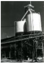
Scoripal Silo's, 1985 (PrLM_026)
