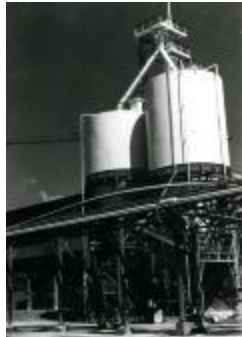
Scoripal Silo's, 1985 (PrLM_026)
